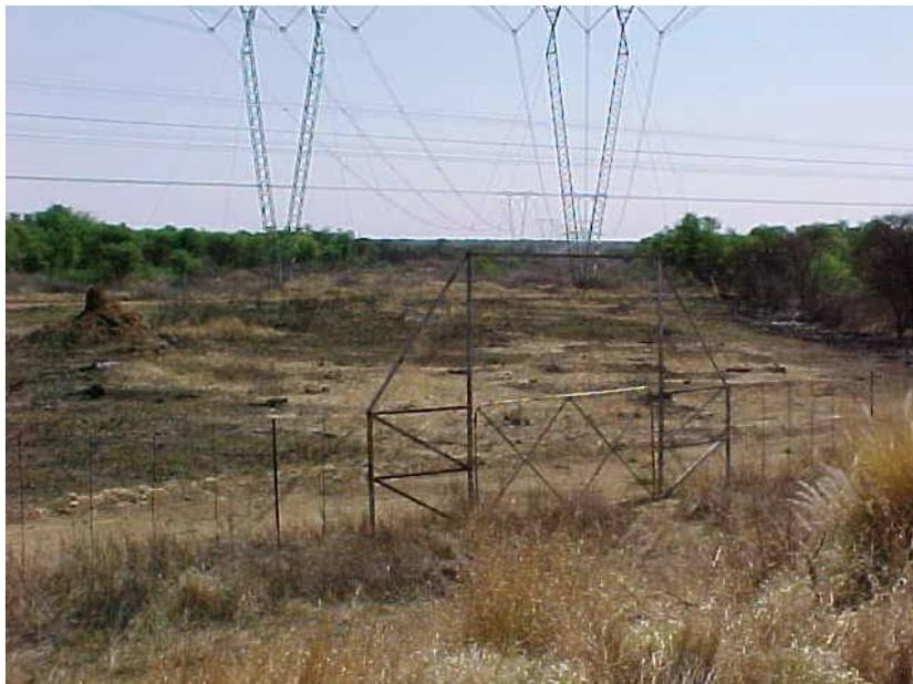
Figure 4 A game fence as used on the Matimba-Spitskop 1&2 lines. Note that the top section has been omitted as per the latest 5m game gate design.
